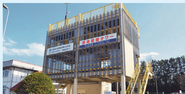
Tsunami evacuation tower.
